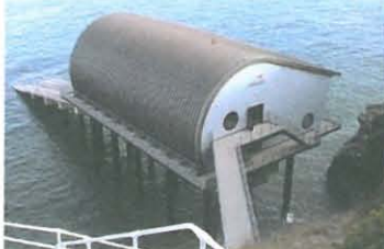
Padstow Lifeboat Station
